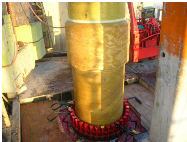
24" Red Box casing being lowered into well
